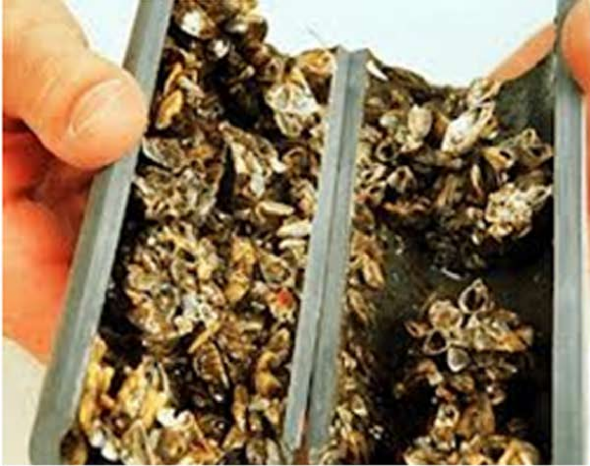
Left photo shows the spread of zebra mussels inside pipe
